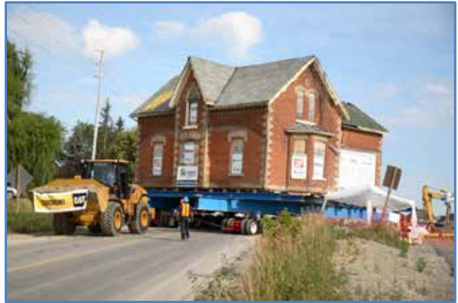
Figure 6.7: Building Relocation
