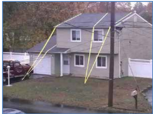
Figure 6.10: Tie-downs for Windproofing
