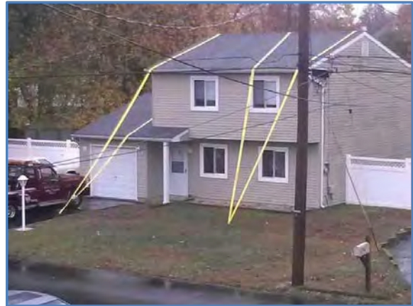
Figure 6.10: Tie-downs for Windproofing
